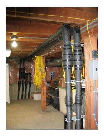
c) Next came the sheet metal work, which was also included in the Lockhart bid. Basically, this company installed all new duct work and venting in the hall as well as connected the duct work to the heat exchange units.
