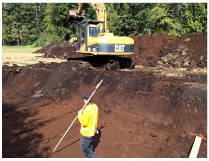
Once the trenching was complete, a small army of volunteers laid the geothermal piping in the trenches and the horse field was then backfilled.
